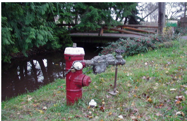
Figure 9: Backflow Prevention Device
