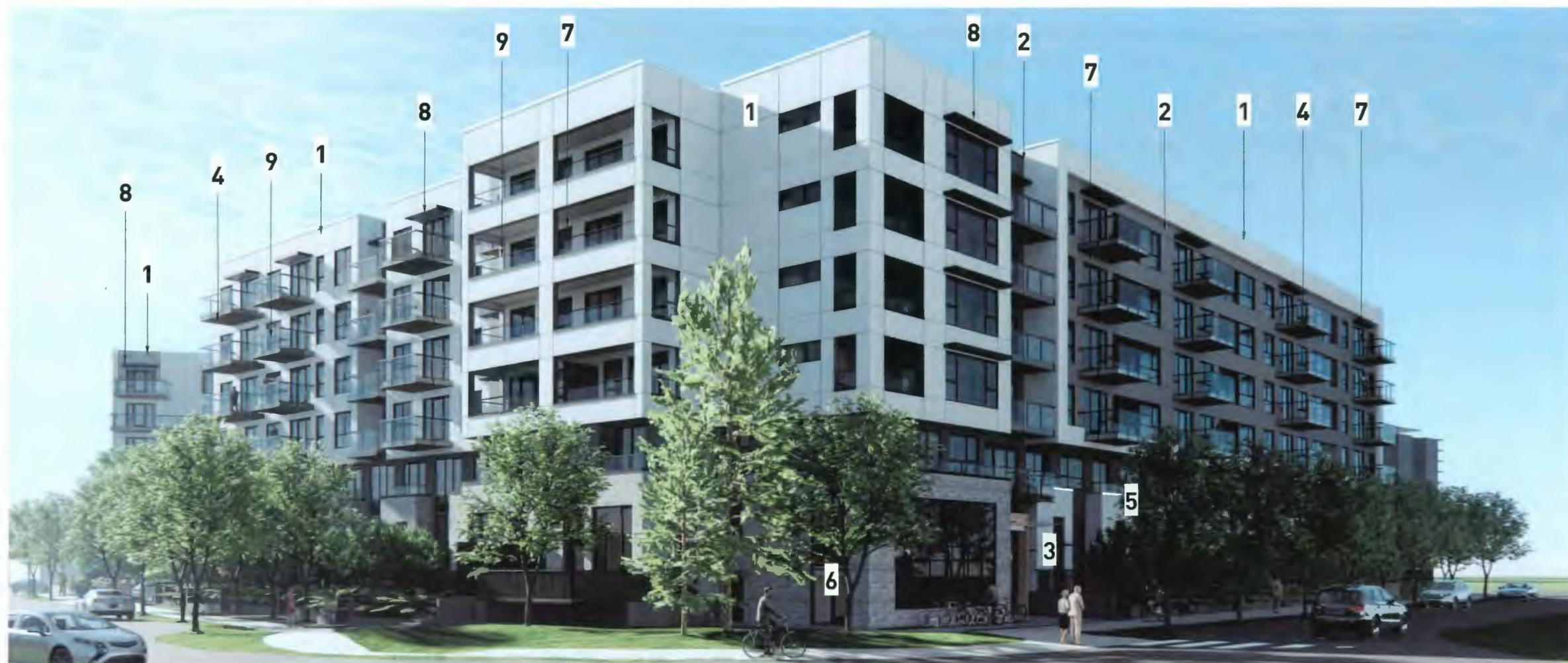
SOUTH WEST VIEW
