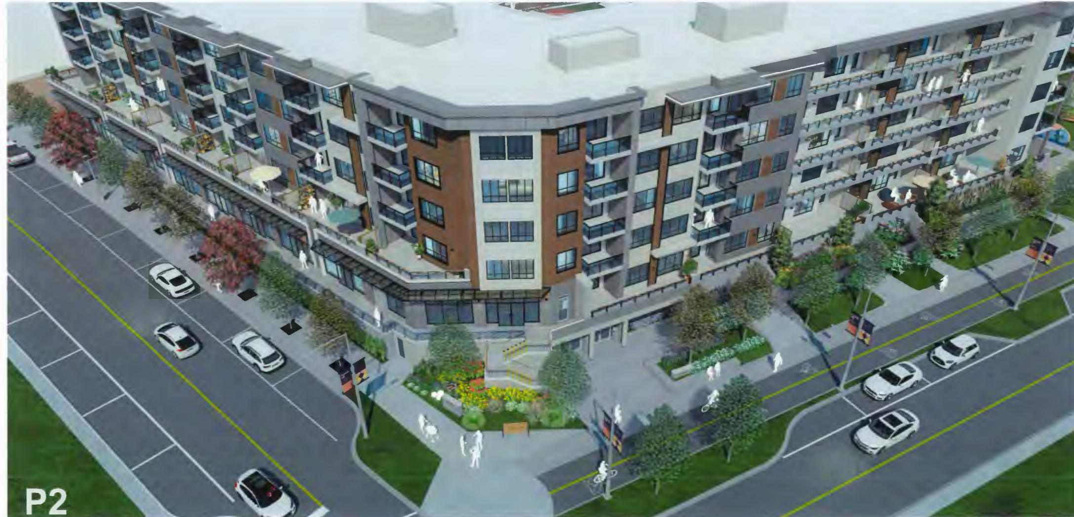
P2 building A - south-east corner view
