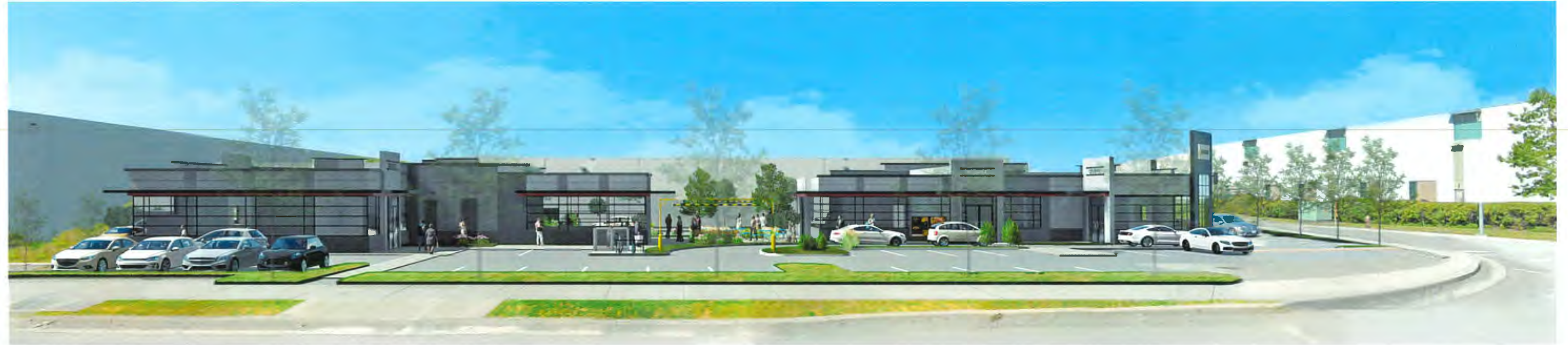
A STREETScape VIEW FROM BLUNDELL ROAD
