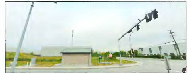
③ VIEW NORTH AT INTERSECTION OF BLUNDELL AND NELSON ROAD
