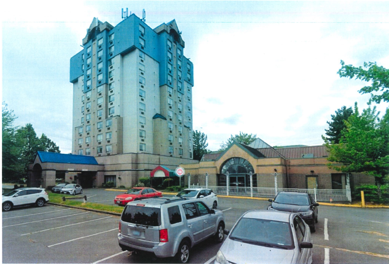
PICTURE OF EXISTING BUILDING
