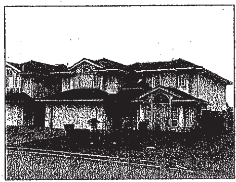
Single-Family housing development
