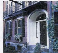
Entry details - planters, rod iron and balconies
