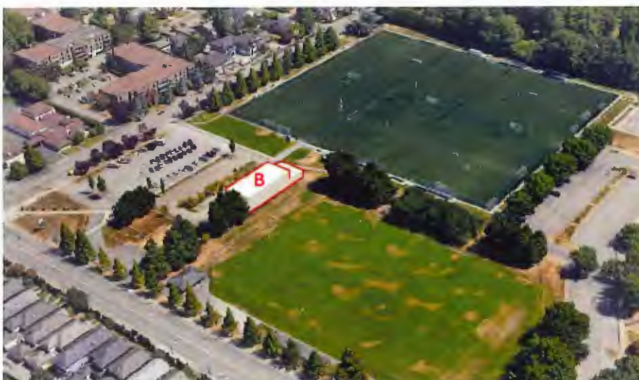
Figure 2: Site B – Aerial View from Northeast
