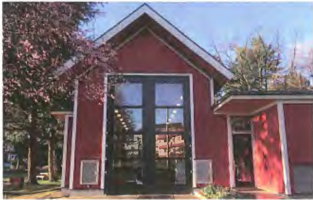
The Interurban Tram building
