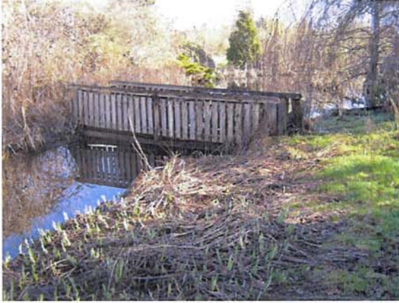
Wooden bridge – The decking and some of the structure needs to be replaced. Recommendation is to remove and replace.
