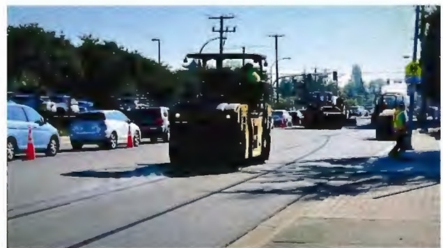
High Recycled Asphalt Pavement Project
