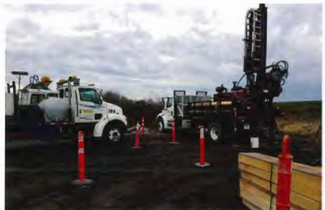
Microbial Induced Desaturation and Precipitation Test
