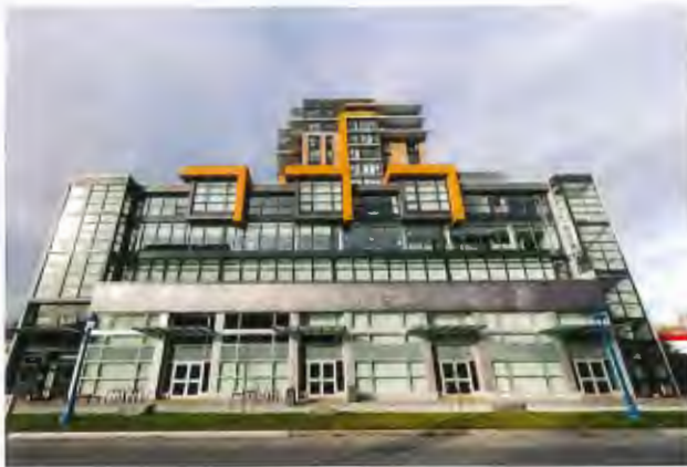
Storeys Affordable Housing Development
