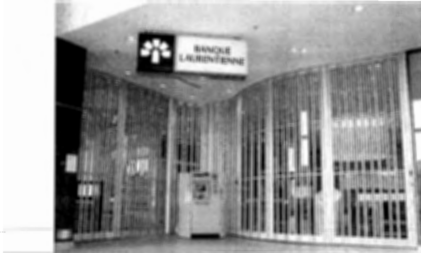
Example of sliding mall dividers to block off ground floor access corridors
