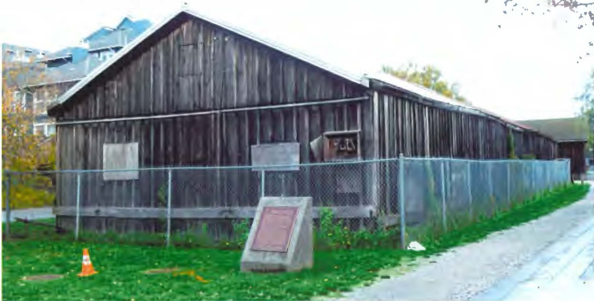
First Nations Bunkhouse at Britannia Shipyards National Historic Site, 2021
