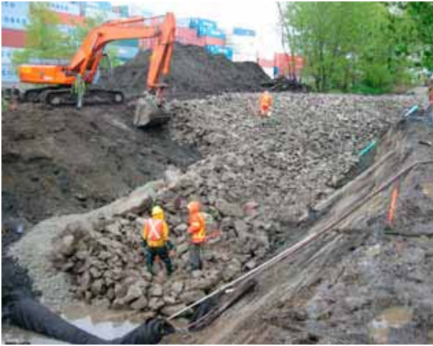
Top Left: Dyke restoration and improvements are an important part of Richmond's long-term flood protection strategy.
