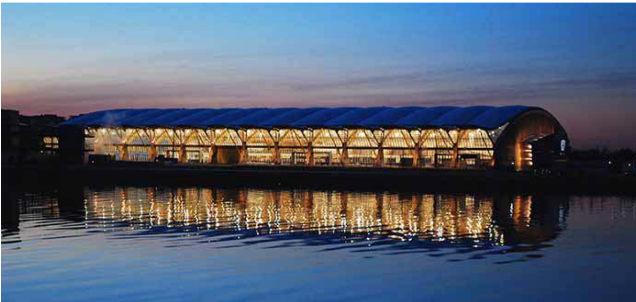
Construction of the Richmond Olympic Oval was completed without raising taxes or external borrowing to finance the project.
