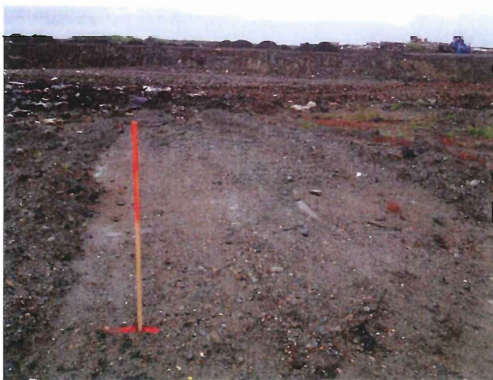
Photograph 2: Fill and final fill elevation in the background for the northern portion of the property proposed for Tervita's operations
