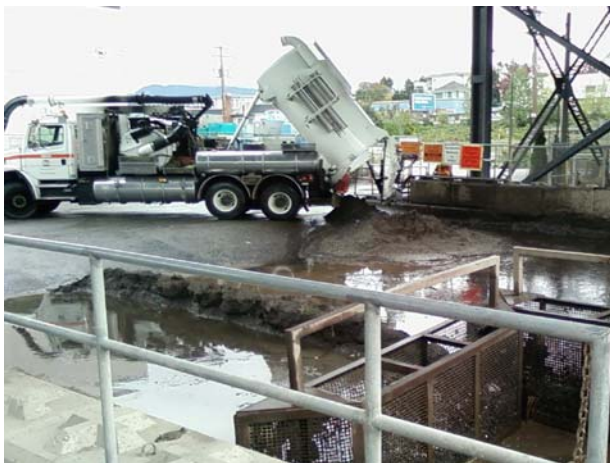
Fig C – Vernon Drive Operation, Vancouver
