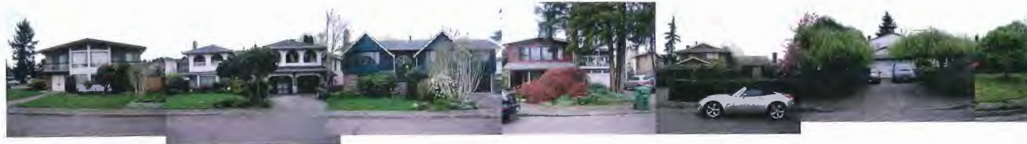
WEST SIDE GOWER STREET
