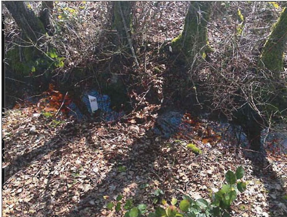
Photo 6. Perimeter ditch on 10880 at property pin (March 2013)
