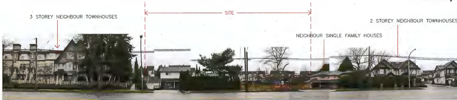
SITE VIEW FROM NO. 1 ROAD
