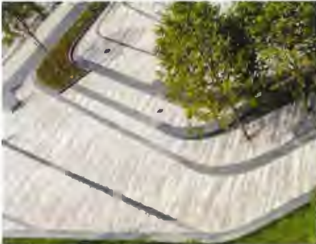
FEATURE UNIT PAVING WITH BANDS
