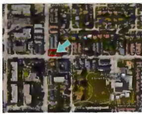
SITE AERIAL PHOTO
