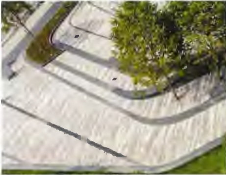
FEATURE UNIT PAVING WITH BANDS
