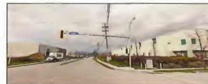
④ VIEW NORTH AT INTERSECTION OF BLUNDELL AND NELSON ROAD
