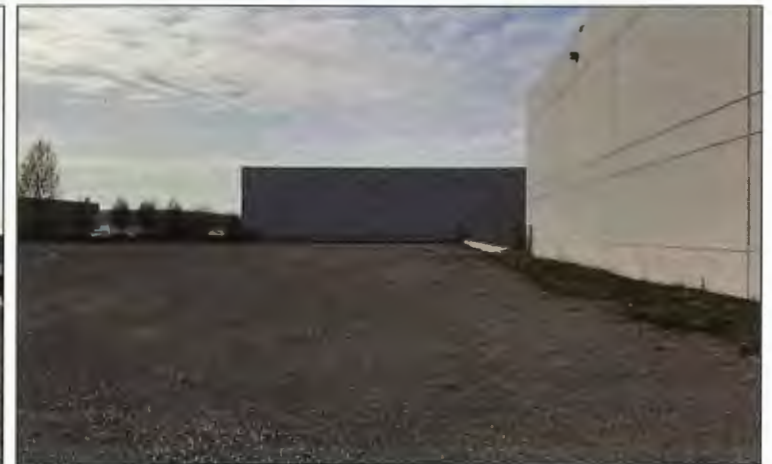
④ VIEW FROM THE SITE LOOKING EAST TO ANIXTER ELECTRICAL BUILDING
