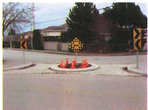
Figure 2: Diagonal Diverter on Ash Street at Dayton Avenue - After
