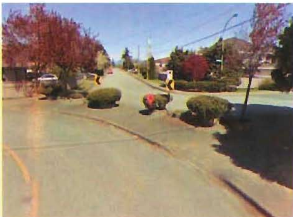
Figure 1: Diagonal Diverter on Ash Street at Dayton Avenue - Before
