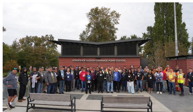
Horseshoe Slough Drainage Pump Station
