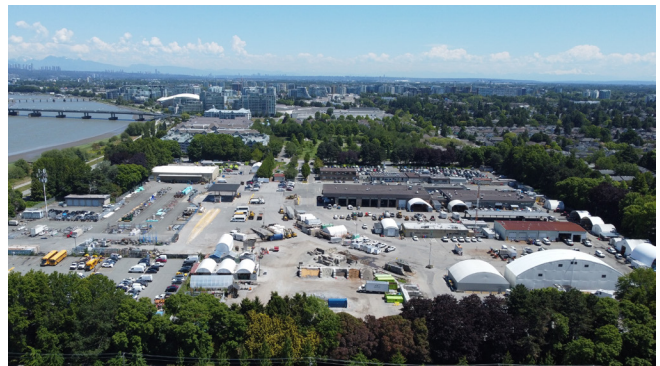
Major Construction Project – Works Yard Replacement Project
