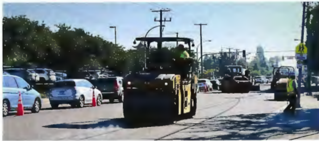
Recycled Asphalt Paving on No. 5 Road
