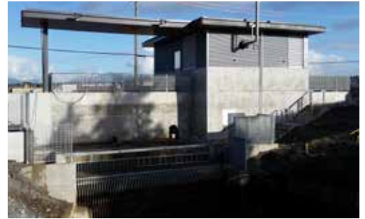
Bath Slough drainage pump station
