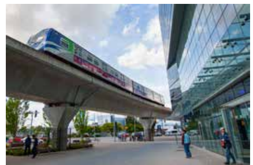
Canada Line on No. 3 Road
