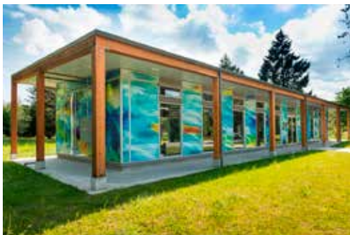
Alexandra District Energy Utility
