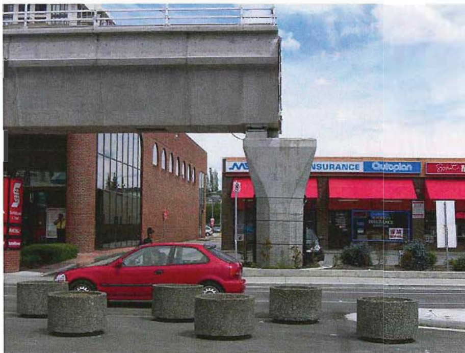
Canada Line terminus guideway and support column, looking East
