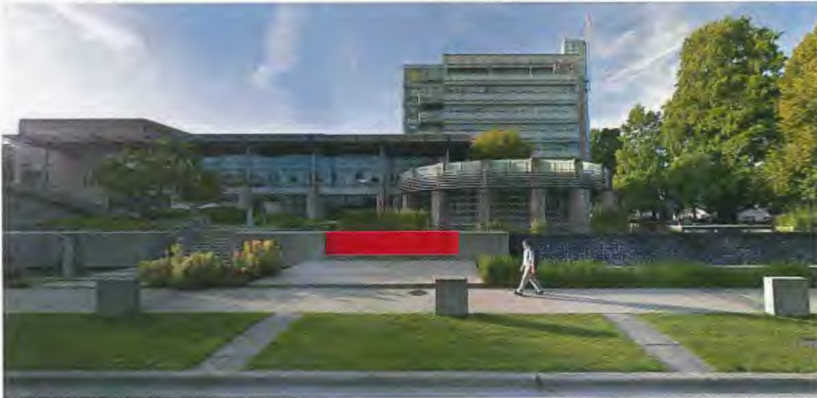
Figure 2 – Concrete retaining wall location highlighted in red.
