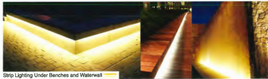
Strip Lighting Under Benches and Waterwall
