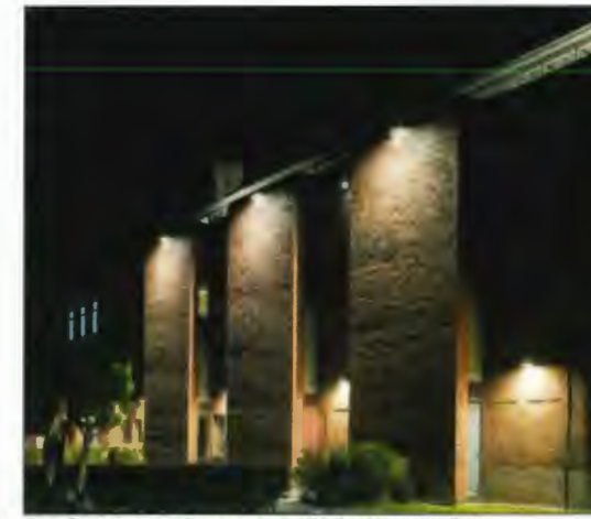
Reference image of down lights grazing facade (Locate similar lighting along top outside edge of "swoop")
