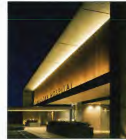
Reference image of Soffit lighting (Locate similar lighting along the soffit of the "swoop")
