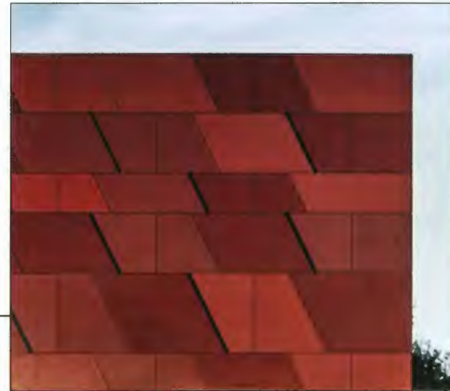
REFERENCE PICTURE - PARKADE ENTRY SOFFIT- FIBER CEMENT PANEL -SWISS PEARL LARGO CARAT - CORAL 7030, 7031, 7032
