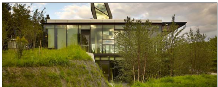
Centre for Urban Ecology, Humber College, Toronto, is designed to integrate with the surrounding ecosystem and result in minimal environmental impact.
