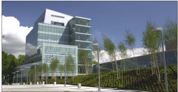
Richmond's City Hall, built in 2000, is a high-performance building that uses natural light to reduce energy use.
