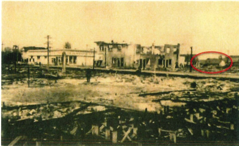
Figure 8: Remaining buildings after the Steveston fire of 1918. Subject site circled. Source: City of Richmond Archives 1978 5
