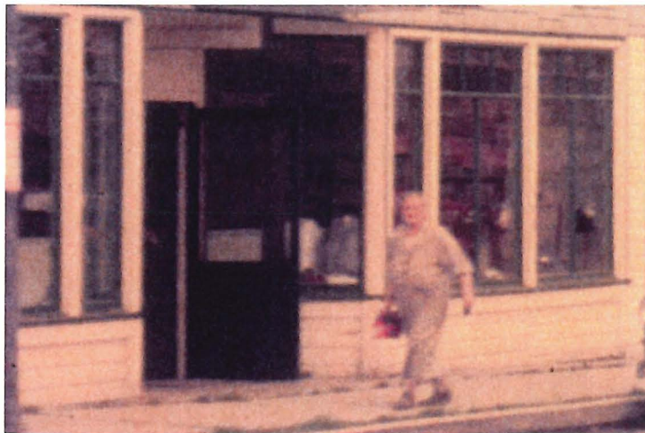
Figure 47: Magnified view of storefront windows and base wall from c. 1950. Source: City of Richmond Archives, Noel McConnell Fonds, Photograph 2012 62b.
