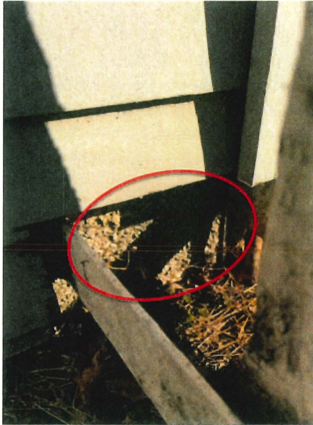
Figure 25: White rock-dash stucco under lap siding (west side, circled)
