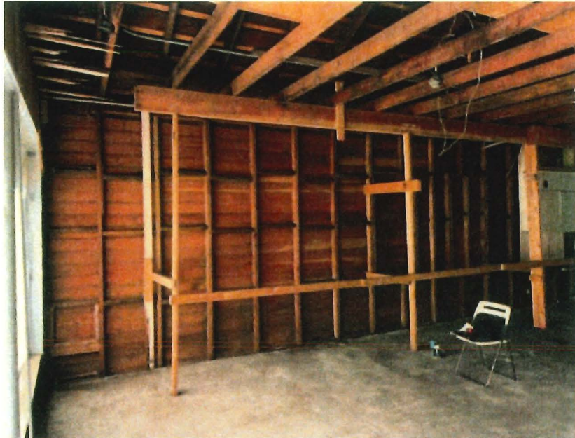
Figure 24: West side wall with back face of cove-cut drop siding intact and visible
