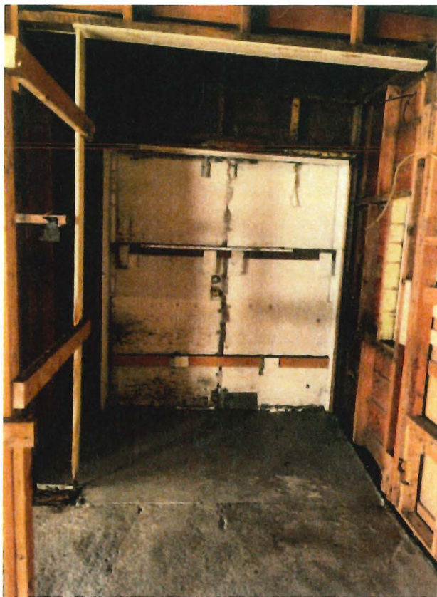
Figure 31: Loading doors on west side as seen from interior, with wall face extended out.
