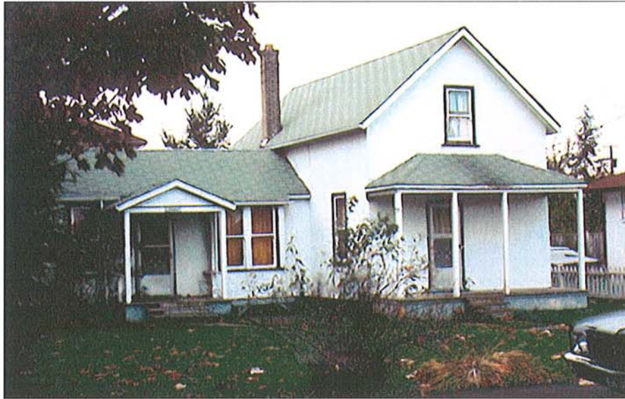
Figure 5. The two Murchison houses in their location on 2nd Avenue shortly before their move to Britannia. (Gordon Kibble photo)
