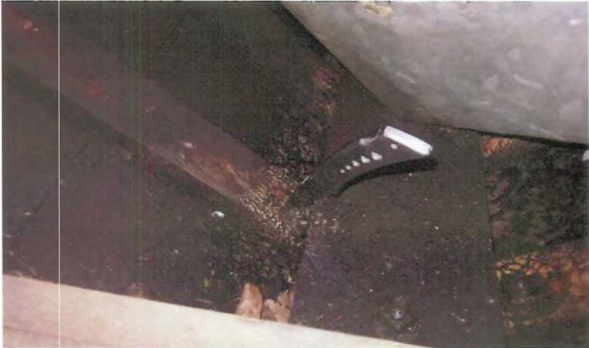
Photo #1 deterioration of rib in forward hull section
