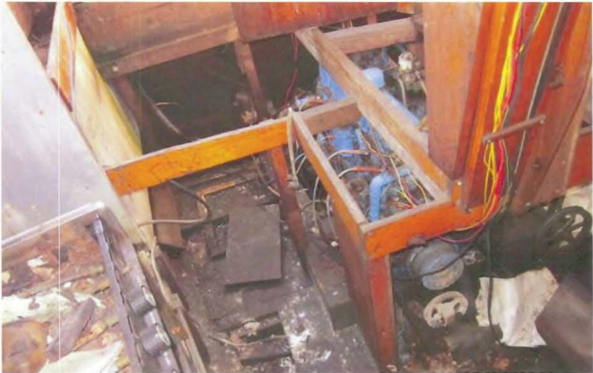
Photo #4 cabin sole broken up note also gasoline engine installation
