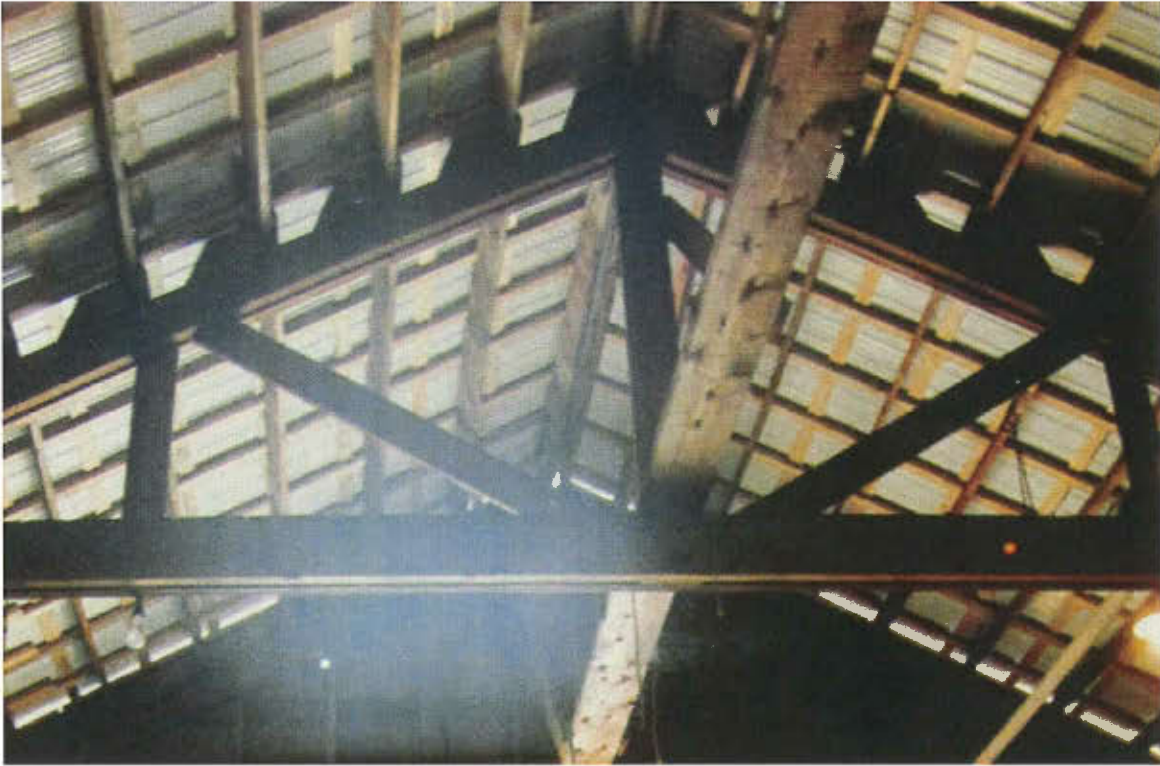
Building #33 interior wood truss, 1984, Existing Building Inspection, Barry Wong
