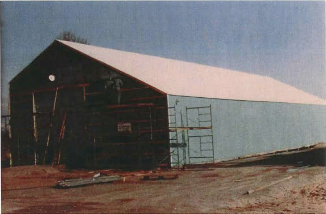
Building #34 with metal cladding being added, 1984, Existing Building Inspection, Barry Wong
