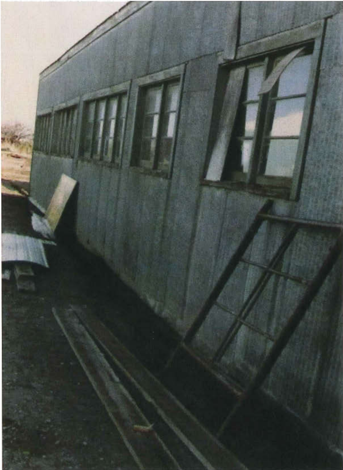
Building #33 windows, 1984, Existing Building Inspection, Barry Wong
