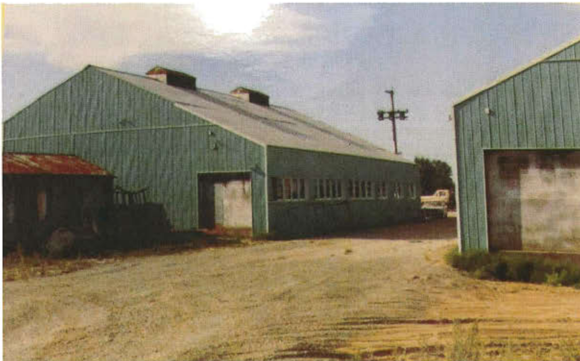
Building #33 with metal cladding, 1984, Existing Building Inspection, Barry Wong
