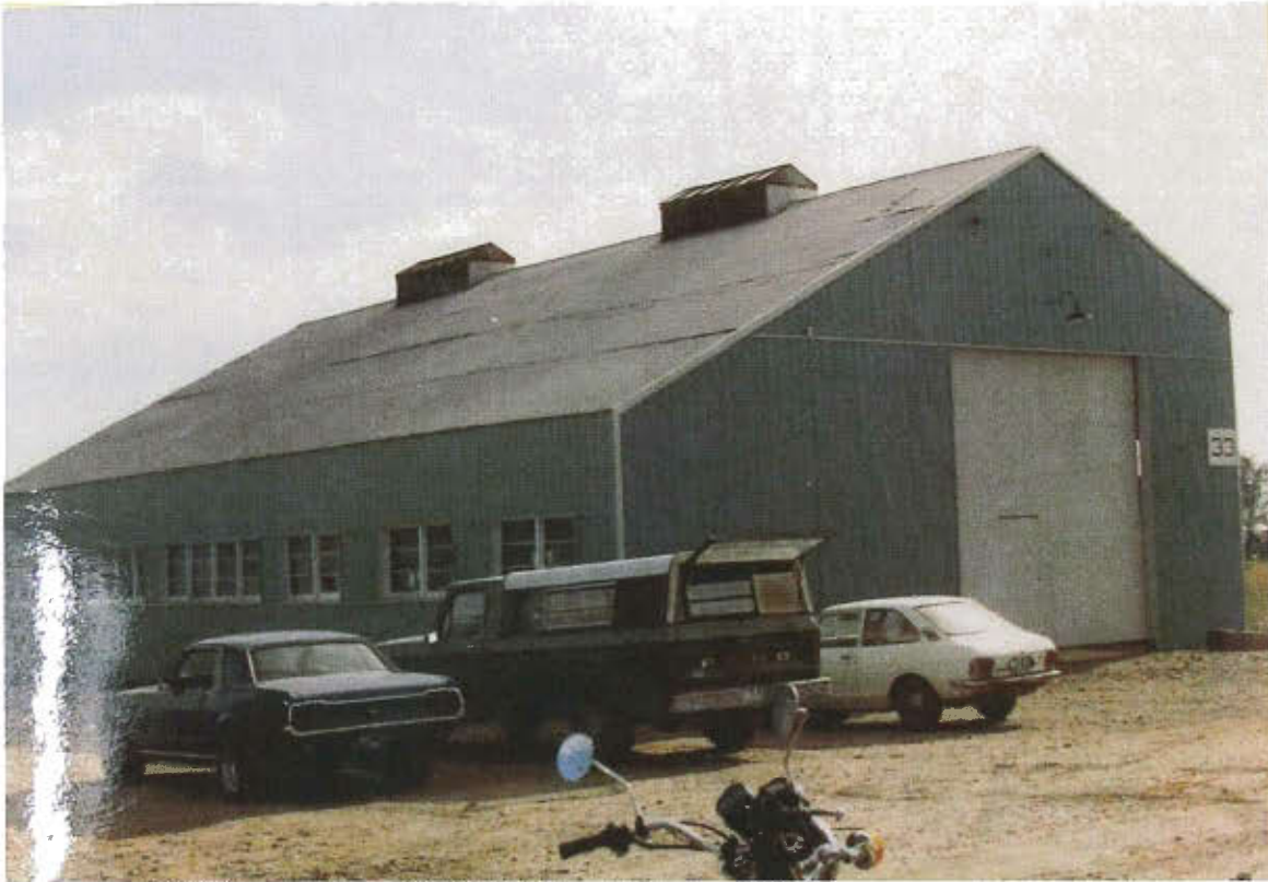
Building #33 with metal cladding, 1984, Existing Building Inspection, Barry Wong
