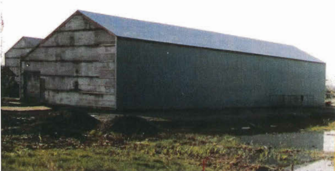
Building #34 with metal cladding being added, 1984, Existing Building Inspection, Barry Wong
