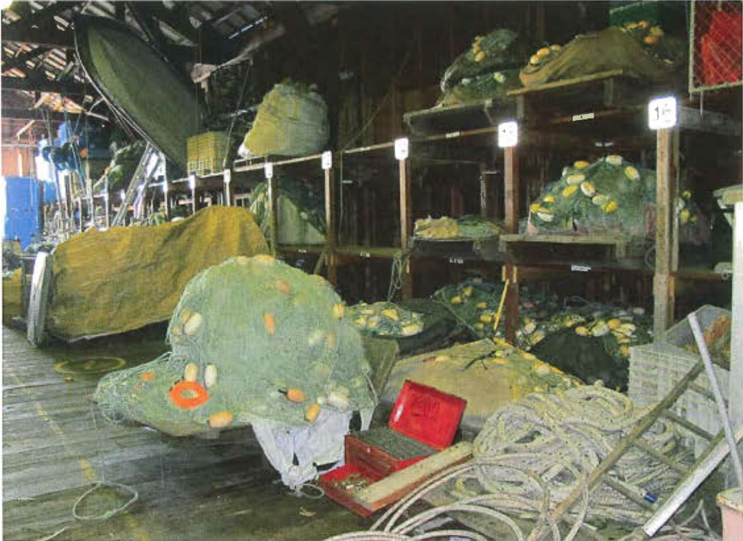
Interior of Building #34 showing floor, storage, wall system and roof trusses, photo taken 2016
