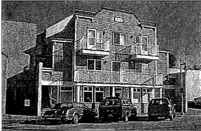
Mixed use development in the Steveston downtown core
