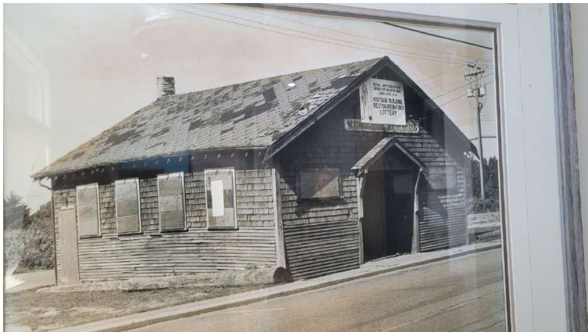
Photograph of the Courthouse building in the office of Oris Consulting. Date unknown. Sign on the building says: "Royal Antediluvian Order of Buffaloes, Lions Lodge No.4 Heritage Building Restoration Fund Lottery".
