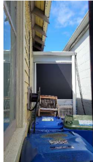
North Side Elevation, behind the gate, showing the connection to the adjacent building
