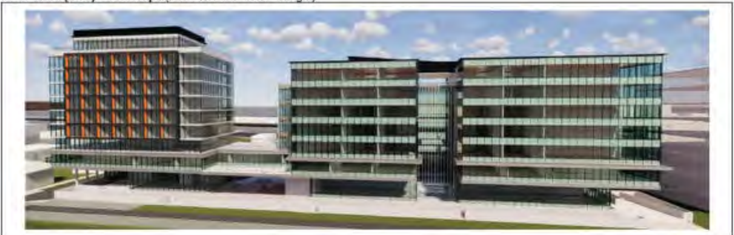
River Road (Dike) Streetscape (Hotel on left & Office on right)
