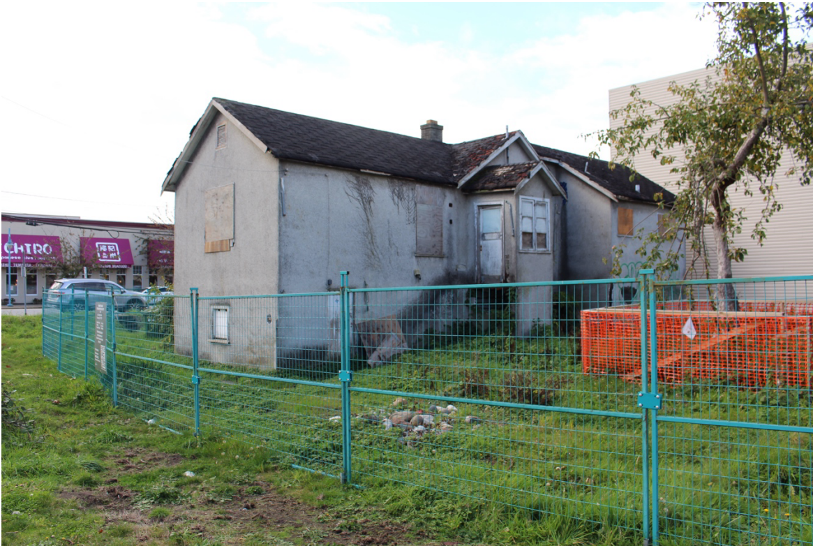
Figure 18: Subject site, house built in 1950 (rear).
