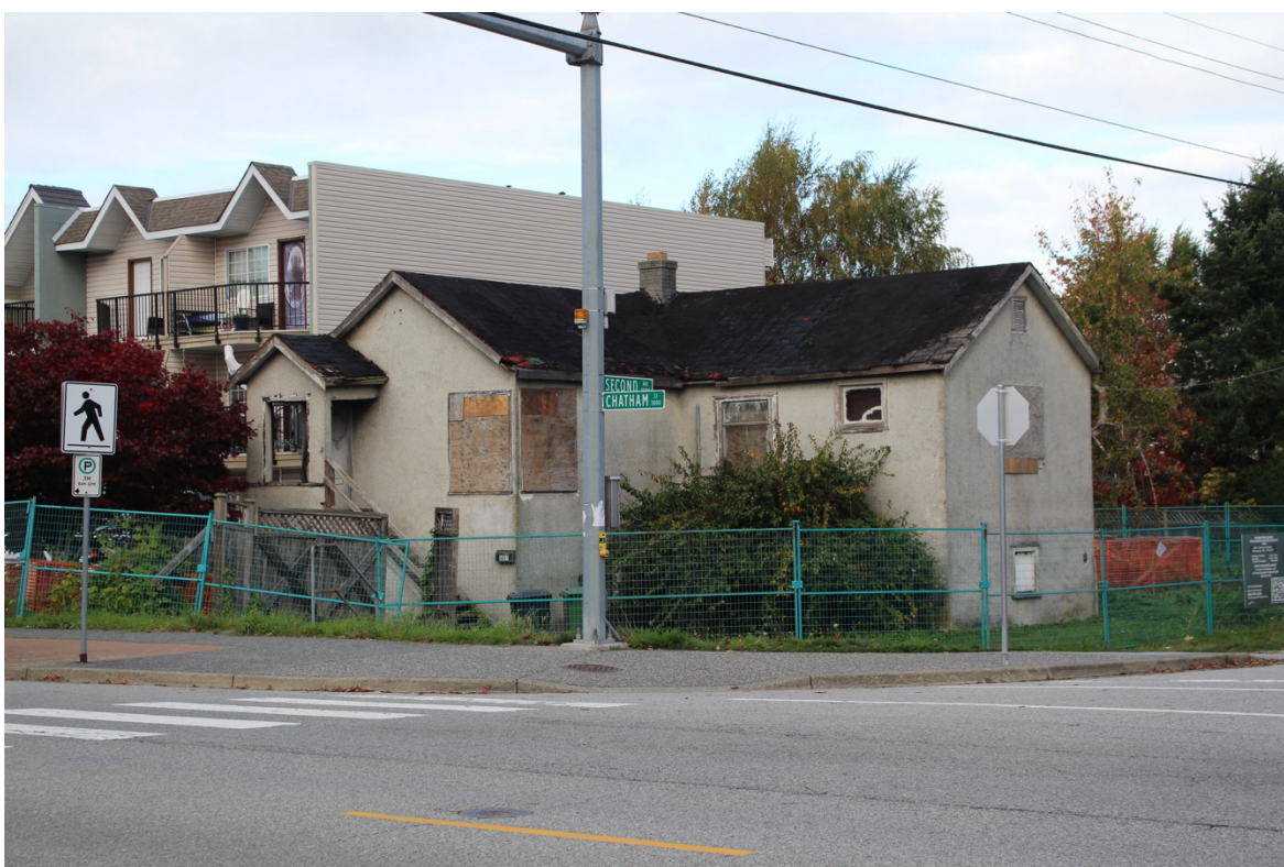
Figure 16: Subject site, house built in 1950 (front and east side).
