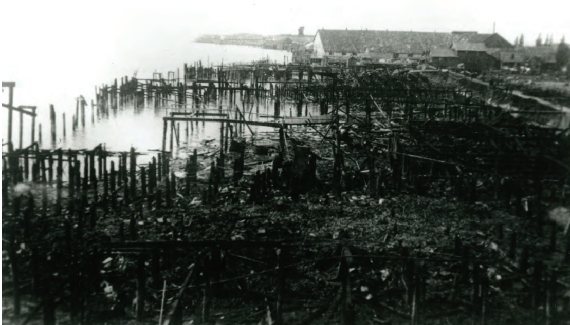
Figure 5: Charred pilings of the Lighthouse, Steveston and Star Canneries after the fire of 1918.
