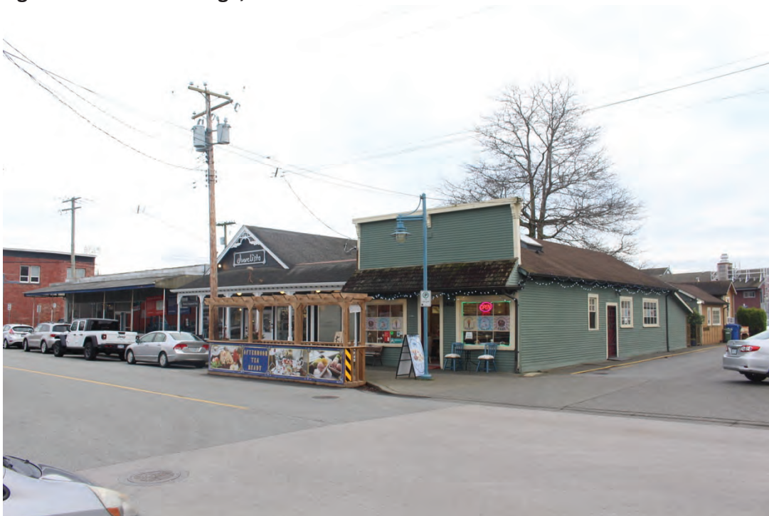
Figure 14: Watsida Building, 3480 Moncton Street (right)
