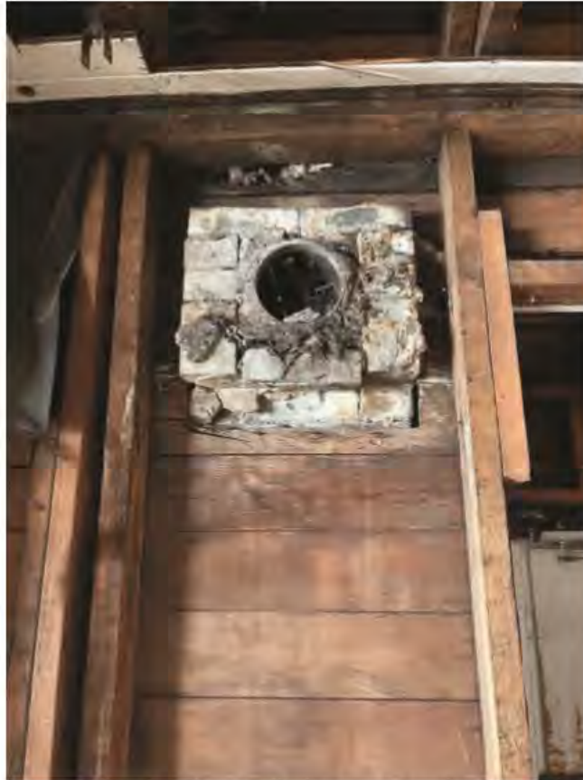
Figure 32: Interior of west wall chimney connection illustrating its original brick form.
