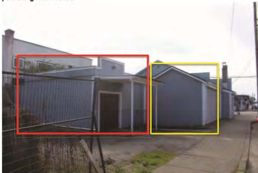
Figure 34: Rear of subject site, with paired recessed loading door facing First Avenue. Earliest addition (c. 1930) outlined in yellow, later addition (1987) outlined in red.
