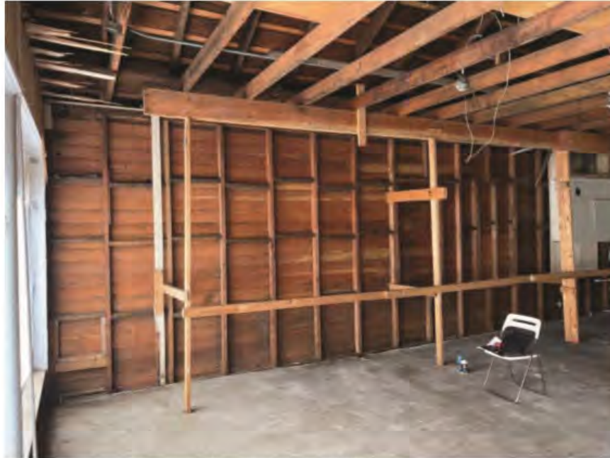
Figure 29b: Broader view of the exposed west side
