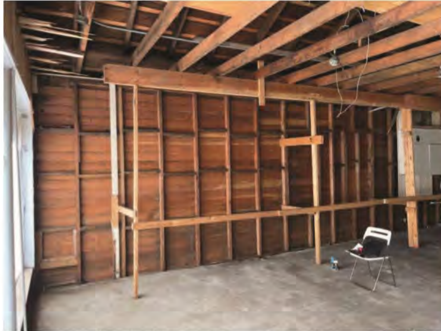
Figure 24: West side wall with back face of cove-cut drop siding intact and visible
