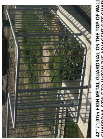
42" / 1.07m HIGH METAL GUARDRAIL ON THE TOP OF WALL, GUARDRAIL STYLE TO MATCH THE ADJACENT SITE GUARDRAIL
