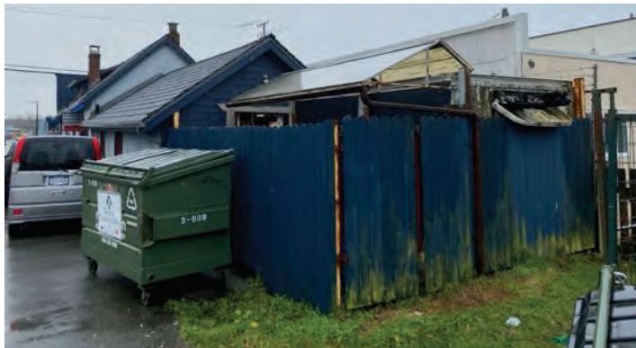
Rear of the building
