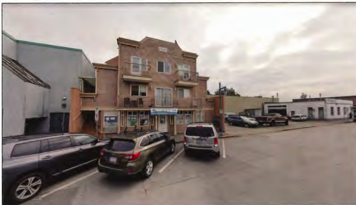
12040 Second Avenue. (Source: Google Street View, 2020)
