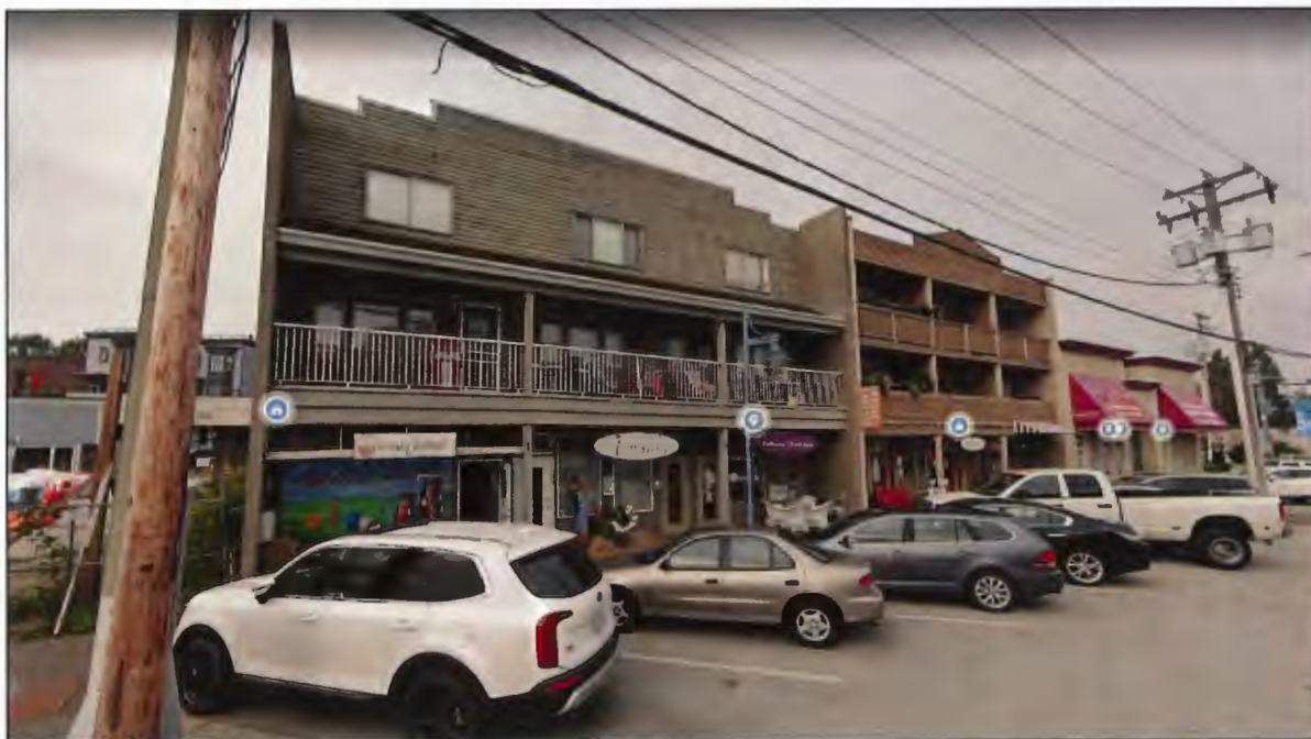
12051 (left) and 12031 (right) Second Avenue. (Source: Google Street View, 2020)
