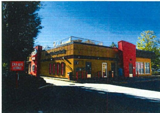
DRIVE-THROUGH EXIT AND EAST FACADE (SOUTHEAST CORNER)
