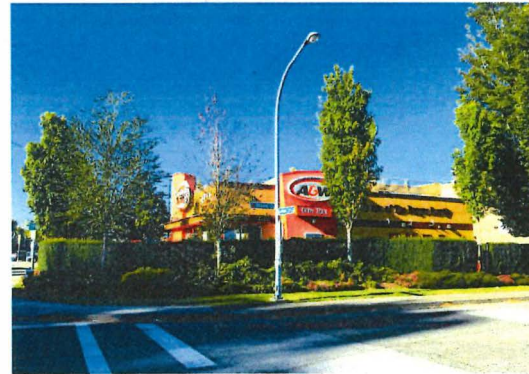
SOUTH FACADE VIEW FROM DIXON AVE (SOUTH)
