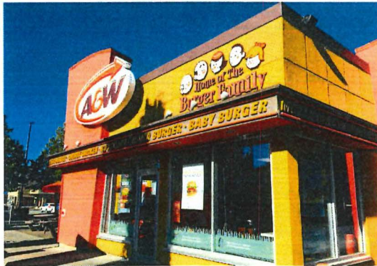
FRONT FACADE (SOUTHWEST CORNER)
