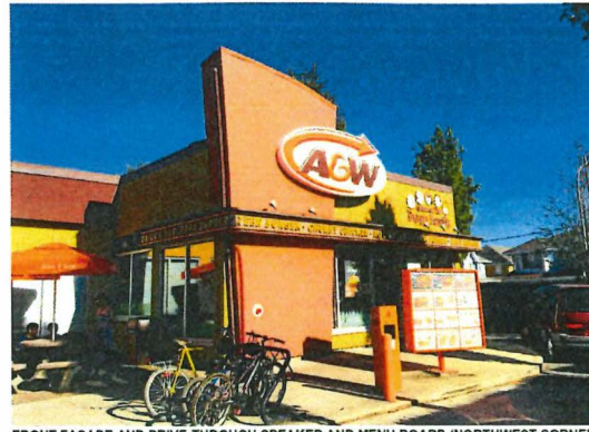
FRONT FACADE AND DRIVE-THROUGH SPEAKER AND MENU BOARD (NORTHWEST CORNER)
