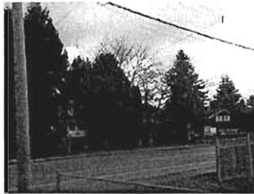
Low overhead wiring at site
