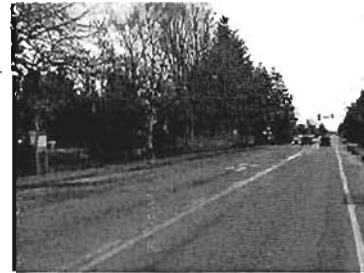
Williams Road looking east
