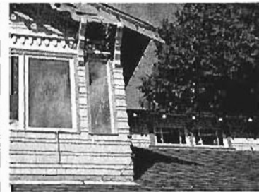
Dormer/upper floor shingle cladding
