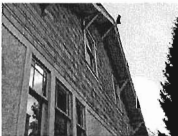
Shingle cladding at side gables
