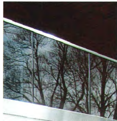
1.2 Glass Guard with MTL-Handrail w/ cont. Base Shoe (no verticals)
