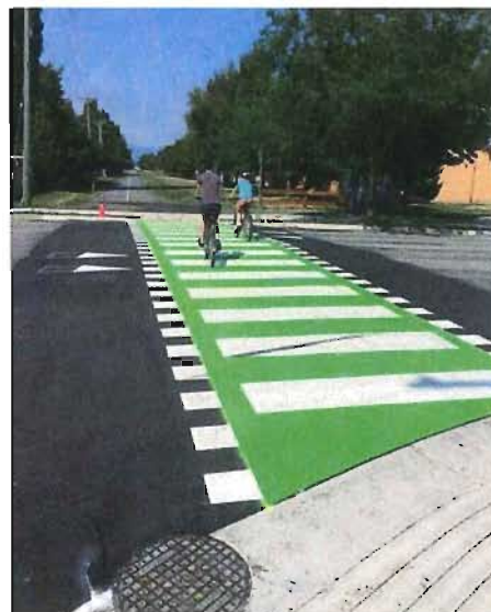
Figure 1: Raised Crosswalk at Granville Avenue
