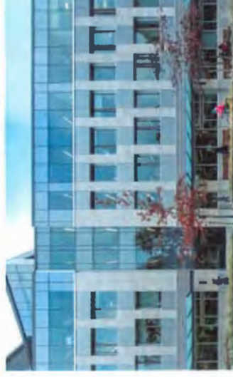
Capital Park, office building, Victoria BC Appropriate window-to-wall ratio with punched windows and less curtain wall areas
