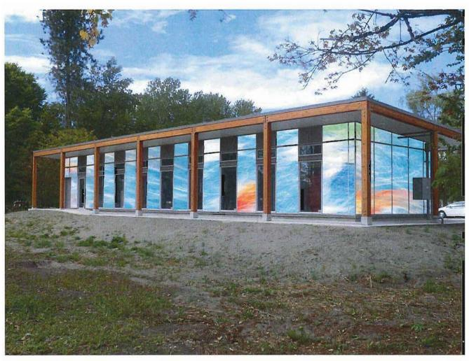
Photographic aluminum panels to be placed over the existing white panels (all sides)
